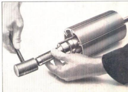
FIG. 7. Fitting the rear ball race on shaft.
