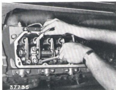
Fig. 25. Adjusting the tappets.
